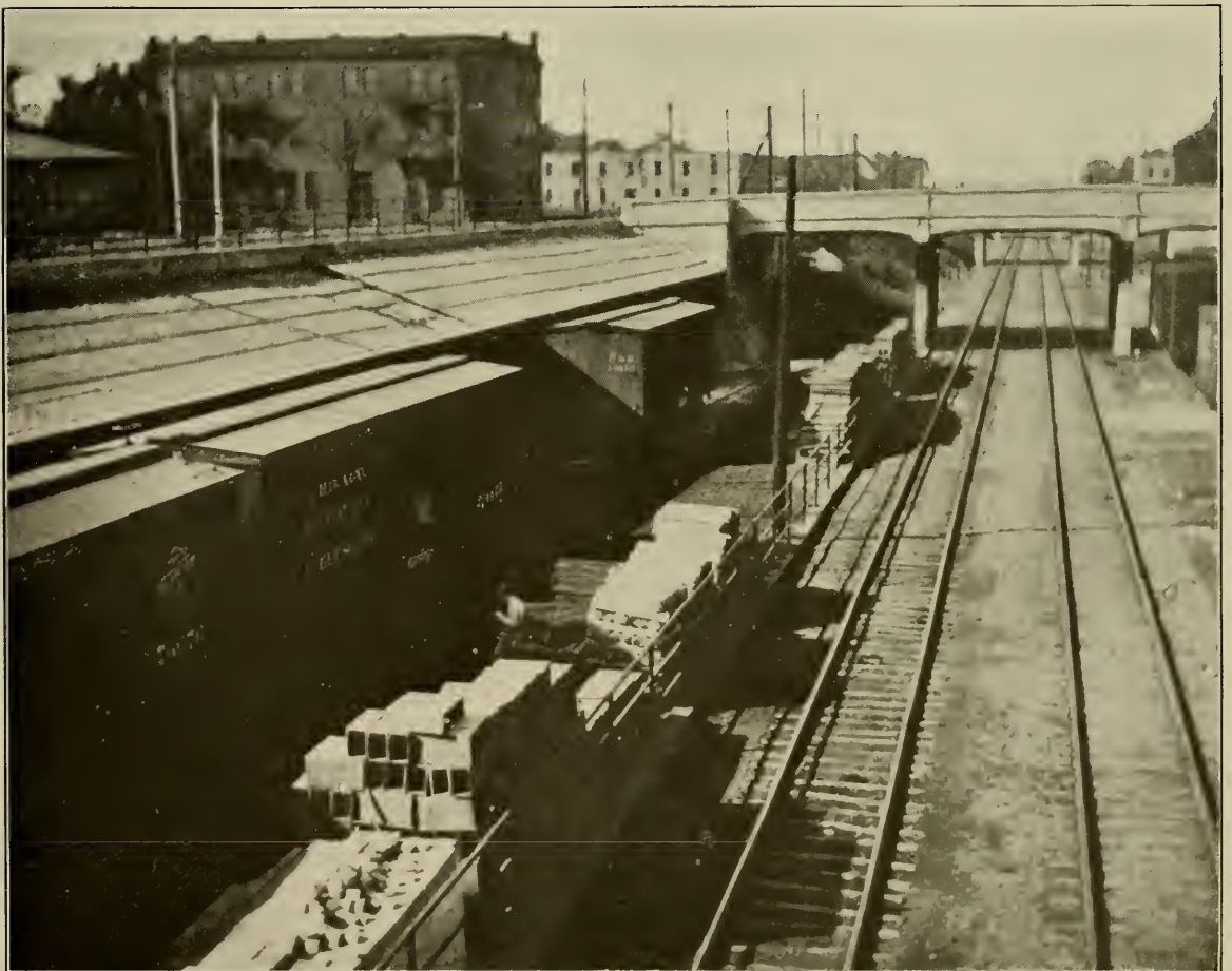
Complete Depression—H. & D. Division, C. M. & St. P. R. R. Minneapolis, Minn. Clearance, 18 feet. Main Line and Industrial Siding.
